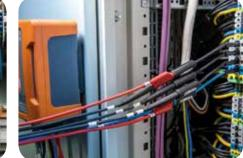
Arrows on all clamps have to be pointed towards the electrical load. • Pay close attention to connecting the analyzer in
